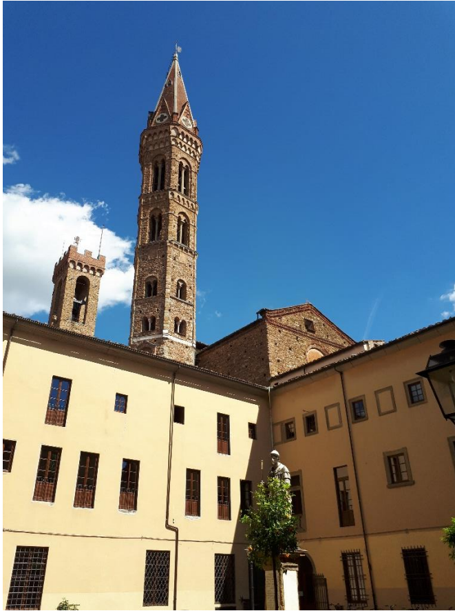
Fig 20 Piazza San Martino, a former convent, now city offices, with the church of Badia Fiorentina in the background
