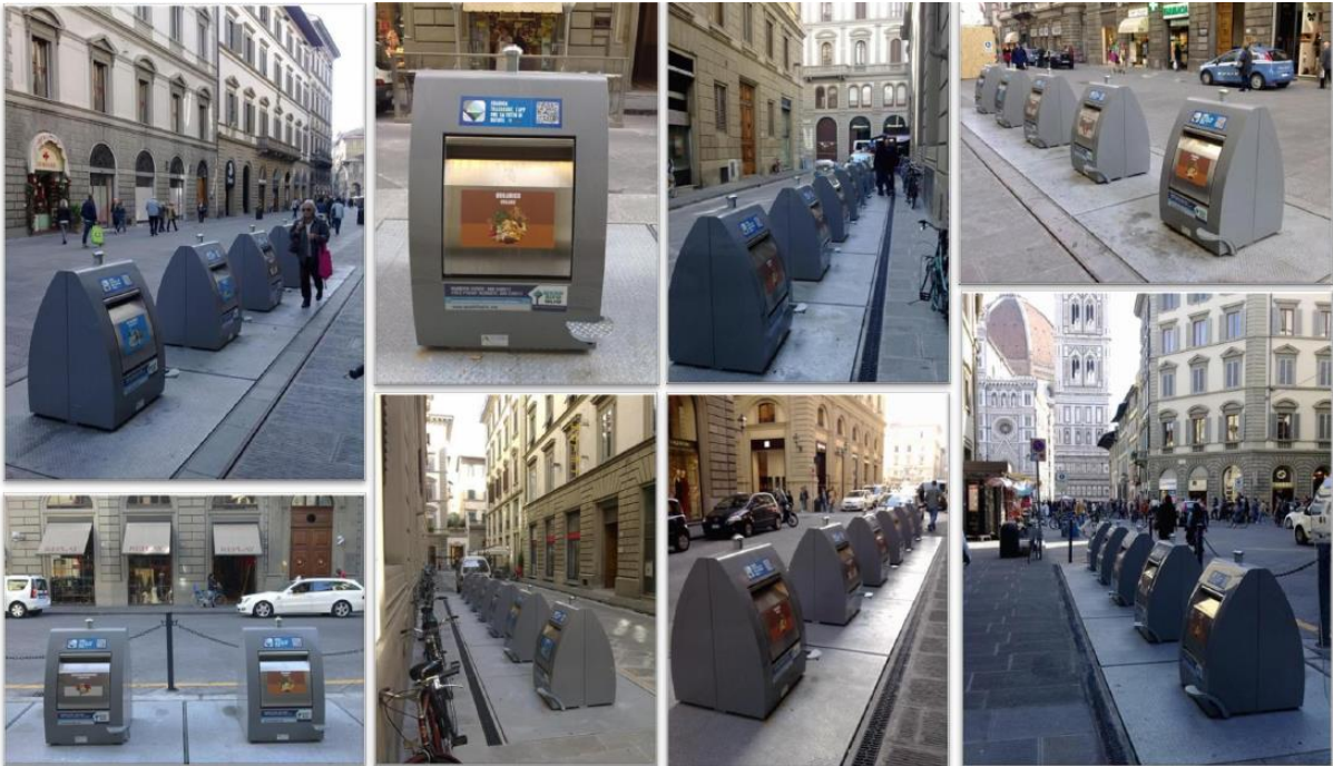
Fig 19 Some underground stations built in the historic centre of Florence
