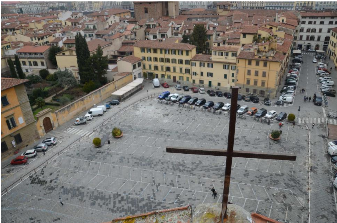
Fig 13 The Nuova Piazza del Carmine from the gable of the Carmelite Church, after removal of most parking; trees will be planted on the far side
