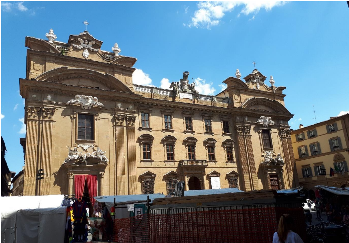
Fig 21 The San Firenze Monumental Complex from the Piazza looking east; the stalls in the foreground are to be removed
